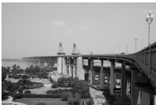
Fig. 10-18 Yangzi River Bridge (Source: http://image.baidu.com/ )
