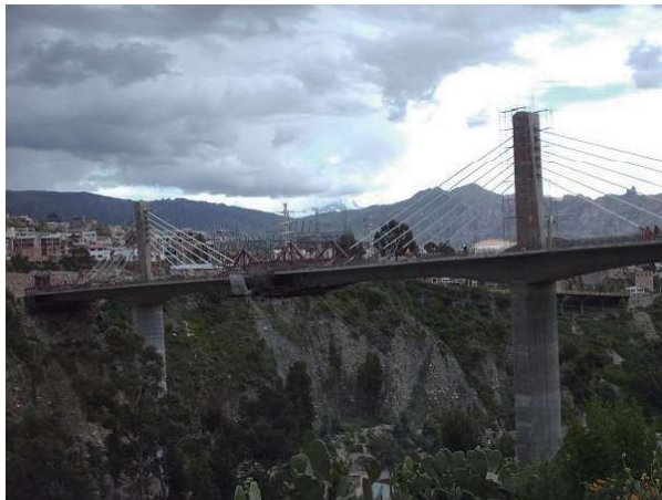
图 1.15 The Triplets Bridge (三兄弟大桥)
