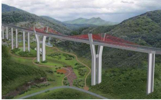
图 1.10 Pyung-Yeo 2 Bridge (平荣 2 桥)
