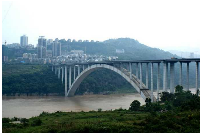
Figure 1.24 The Wanxian Yangtze River Bridge.
