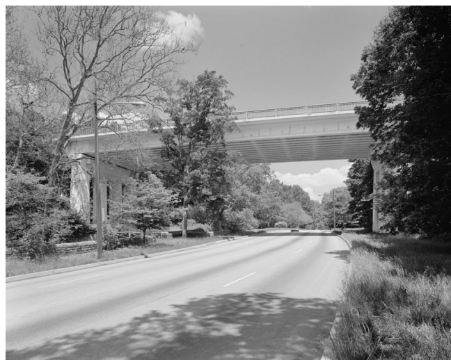
Figure 1.15 The first major prestressed concrete bridge in USA – the Walnut Lane Memorial Bridge.
