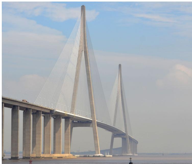
Figure 1.17 The Sutong Yangtze River Bridge, China.
