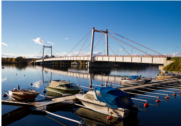
Figure 1.16 The first modern cable-stayed bridge–Strömsund Bridge, Sweden.
