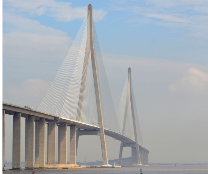
Figure 1.26 The Sutong Yangtze River Bridge, China.
