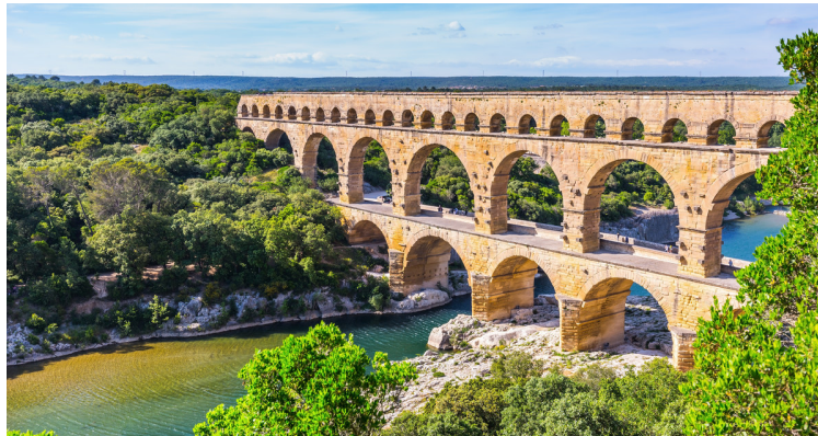
Figure 1.13 The Pont du Gard Aqueduct, France.
