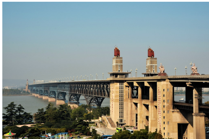
Figure 1.21 The Nanjing Yangtze River Bridge, China.
