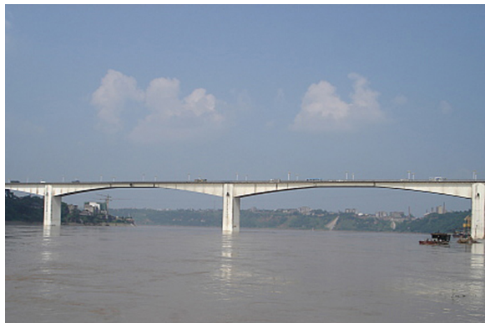
Figure 1.22 The Luzhou Yangtze River Bridge.
