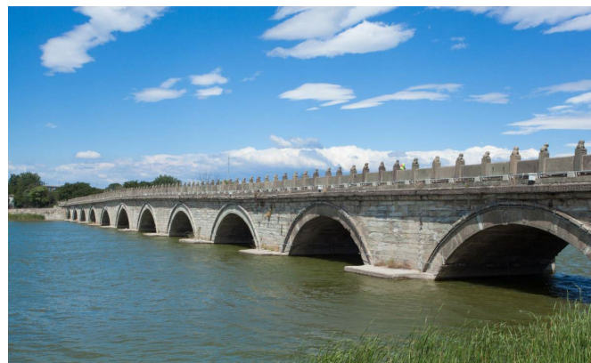
Figure 1.19 The Lugou Bridge-an ancient multi-span stone arch bridge, China.
