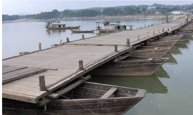
Figure 1.11 A floating bridge.
