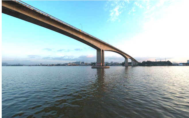
Figure 1.23 The Luoxi Bridge.
