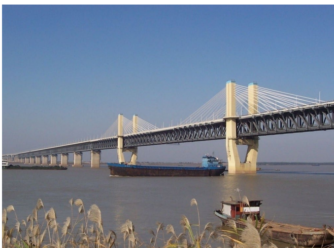
Figure 1.25 The Wuhu Yangtze River Bridge.
