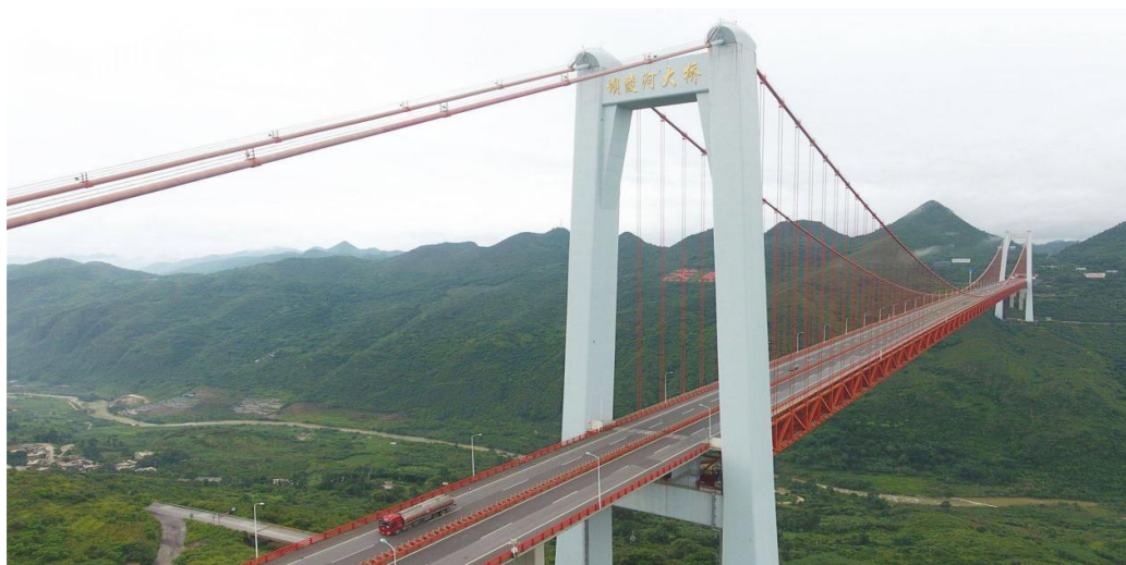
(a) 坝陵河大桥
